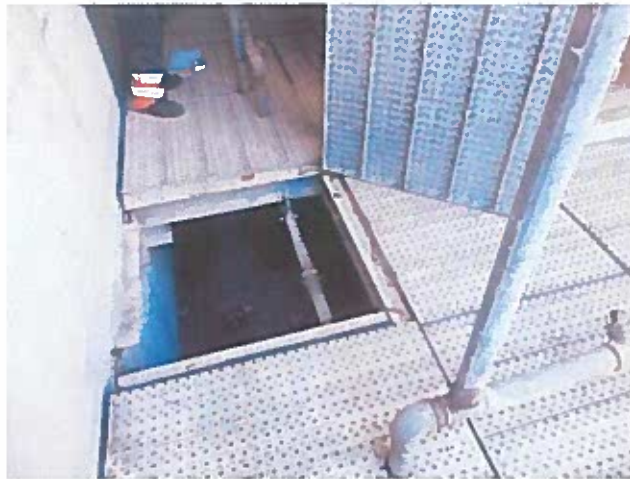
Oil Filled Auxiliary Transformer Bund wall below gratings
